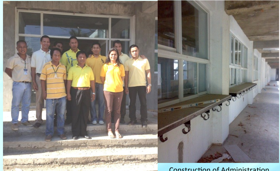
Construction of Administration Building Phase IV
