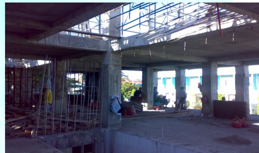
Construction of New Administration Building Phase VI
