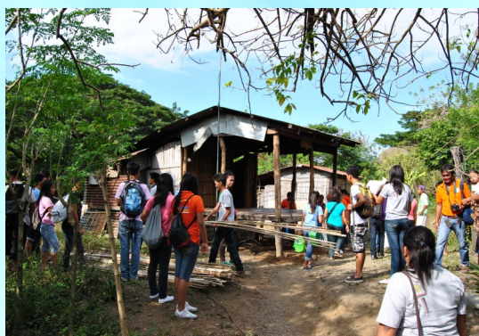
Consolidated effort of UNPians during the repairing process was caught by the camera lens. Working hard for the others at its best.
