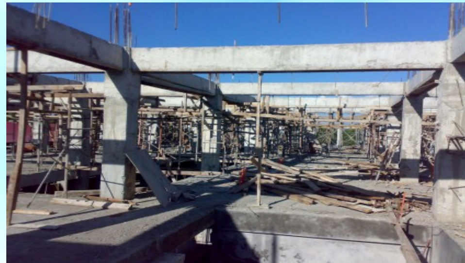
Construction of New Administration Building Phase V
